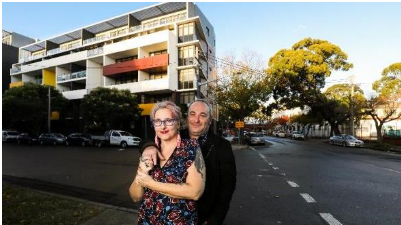
Affordable housing on Hansard Street, Zetland
